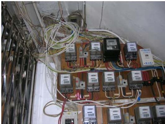
Fig. 2: Individual electrical meters
