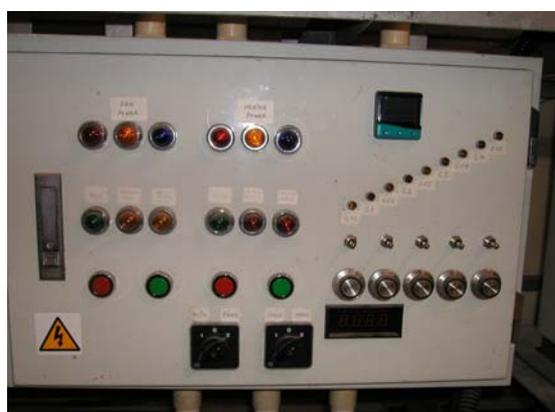
Fig. 7: The PID controller after installation
