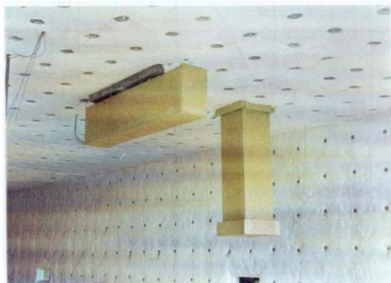
**Fig. 6: Beam and column protected with Vicuclad**
